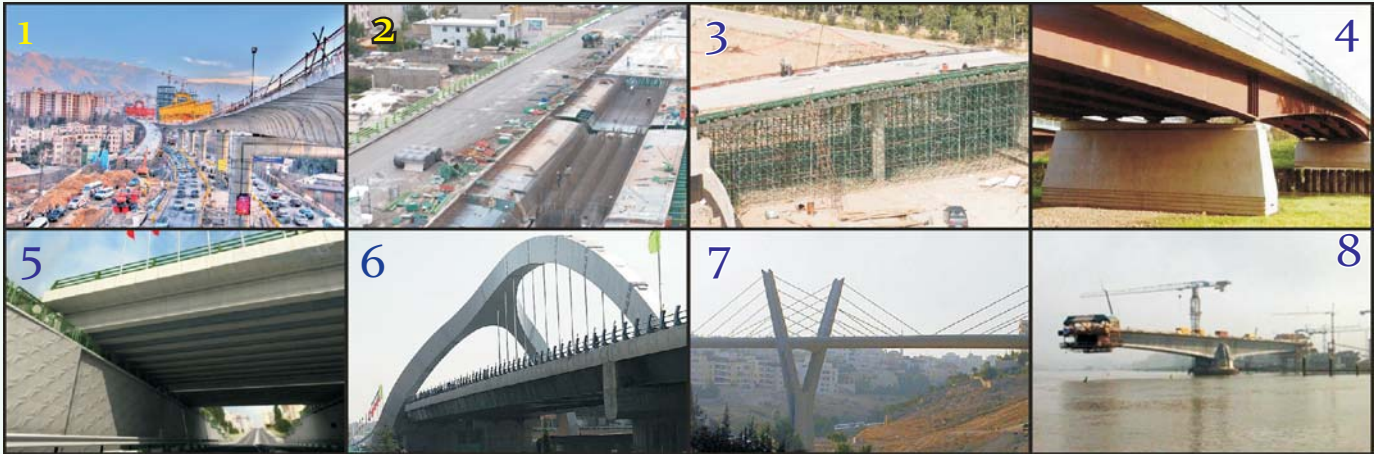
Figures: (3-10): 3- Sadr Elevated Expressway, Under Construction (2012), Tehran, IRAN; 4- The Vafadar Bridge, Constructed (2012), Tehran, IRAN; 5- Abbaspour University Box Girder Bridge, Constructed (2012) Tehran, IRAN; 6- Steel Multi-girder bridge using variable depth girders Westgate bridge, Gloucester; 7- Sazman Aab Bridge, Constructed (2008), Tehran IRAN; 8- : Javadieh Bridge, Constructed (2010), Tehran, IRAN; 9- Abdoun Bridge, Constructed (2006), Amman, Jordan; 10- Pierre Pflimlin bridge being built over the Rhine south of Strasbourg
